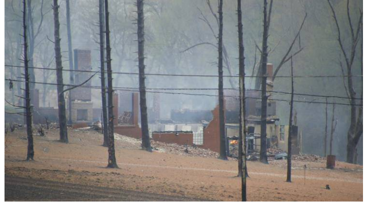
A Salem Township, PA home destroyed by a 30-inch pipeline explosion on April 29, 2016. Keith Srakocic AP photo.
