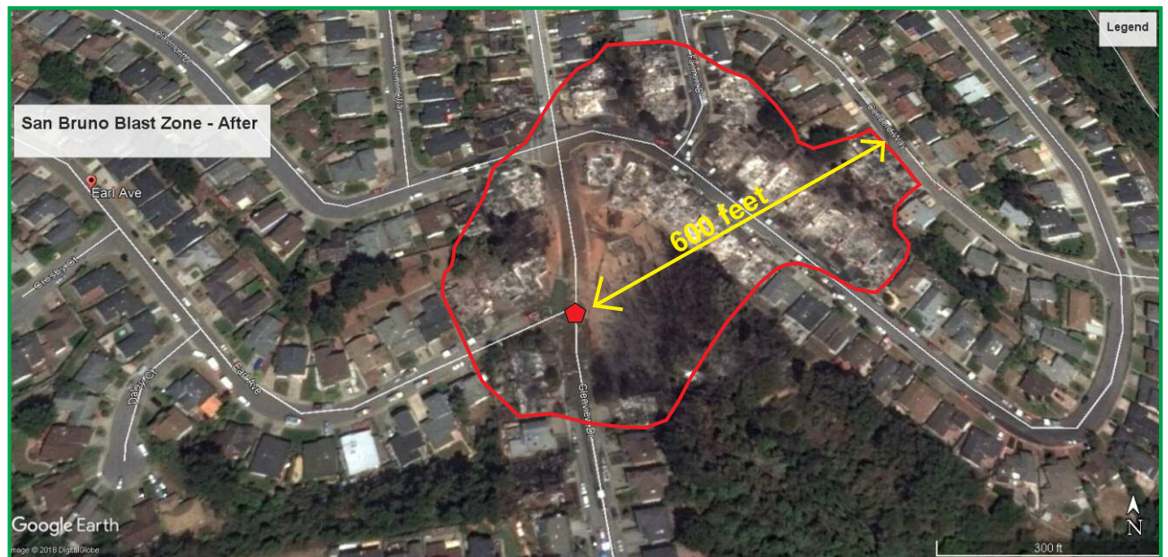
Red polygon: ~Blast zone with homes leveled on Sept. 9, 2010. Google Earth photos.
