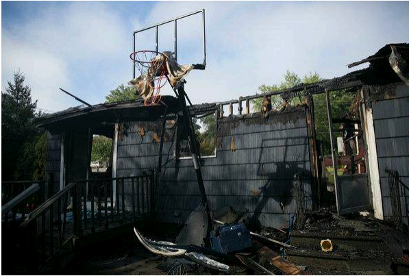
A destroyed home in Lawrence, MA on Sept. 13, 2018. As many as 40 buildings were burned due to a natural gas explosion. Katherine Taylor for the New York Times
